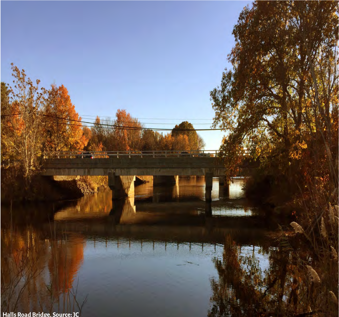
Halls Road Bridge, Source: JC
