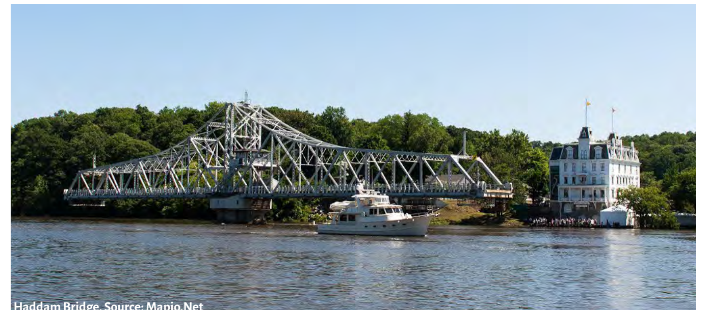
Haddam Bridge. Source: Mapio.Net
