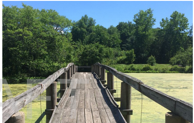
Bridge on Westlake Trail in Middletown in need of repairs Source: RiverCOG
