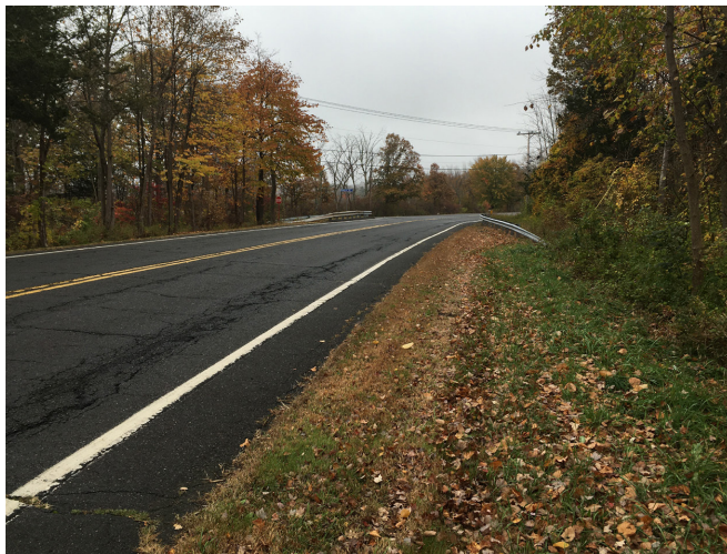
Narrow shoulder on Route 17 in Durham Source: VN Engineers, RiverCOG
