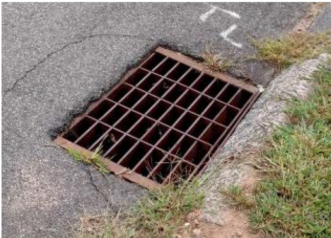
Non-bicycle friendly grainage grate identified during the 2016 RSA Source: Main Street (Route 99) Road Safety Audit
