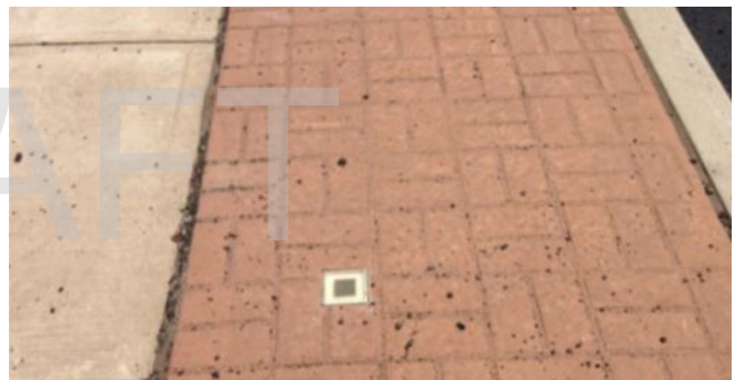
Decorative pavers and lighting installed as part of the streetscape improvements on Main Street Source: Portland Road Safety Audit, 2016
