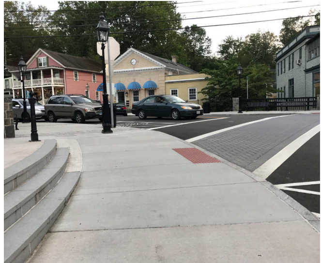
ADA compliant crossing as part of the sidewalk enhancement project in Downtown Chester. Source: FHI Studio
