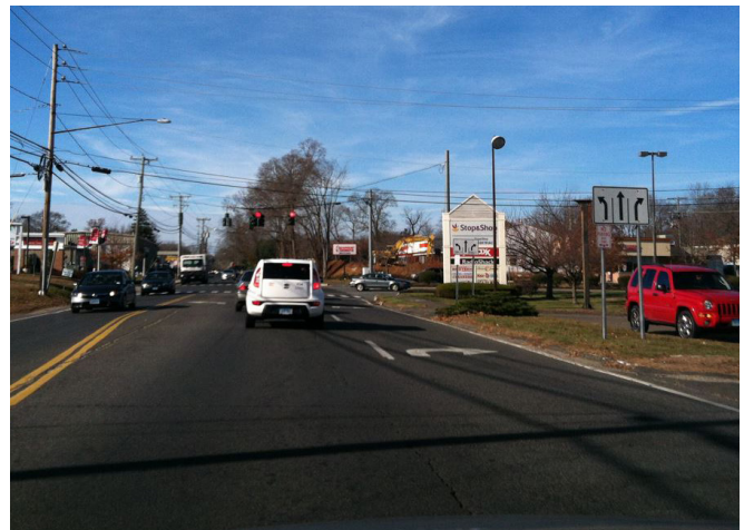
Lack of sidewalks in a commercial area of Route 1 in Clinton Source: FHI Studio
