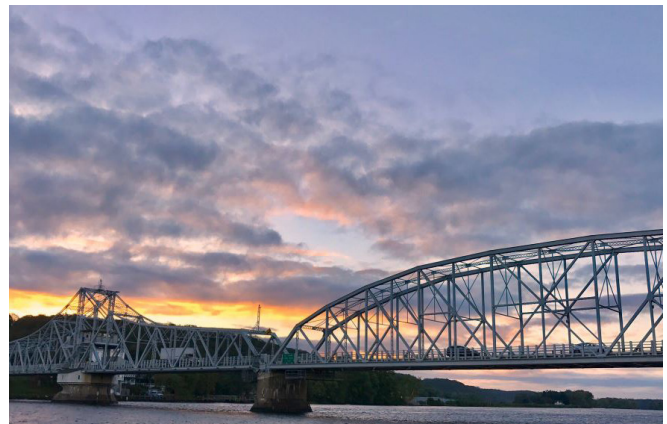
East Haddam/Haddam Swing Bridge Source: RiverCOG
