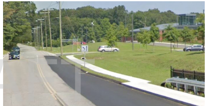
Sidewalk installation on Route 81 near the High School Source: FHI Studio
