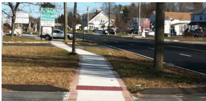
Sidewalk with tactile warning strips on Route 1 in Old Saybrook Source: FHII Studio
