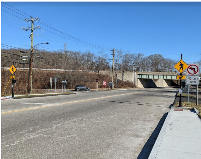
Rectangular Rapid Flashing Beacon recently installed in Essex Note: crosswalk had not yet been striped at time of photo taken January 2022 Source: FHI Studio
