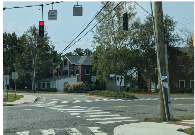
Intersection crossing upgrades in Centerbrook Source: FHI Studio
