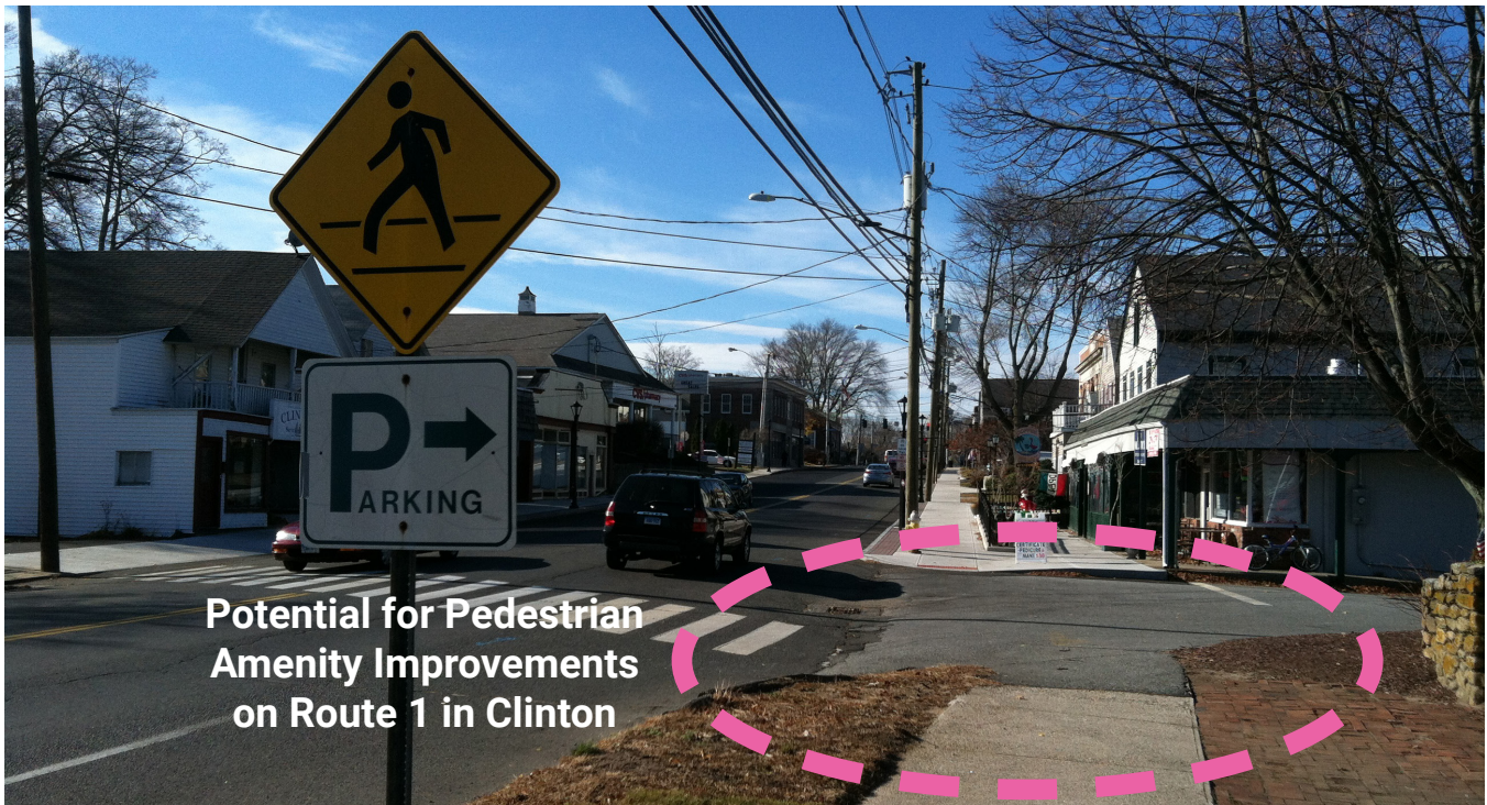
Missing crosswalk and ADA Ramp on Route 1 in Clinton Source: FHI Studio
