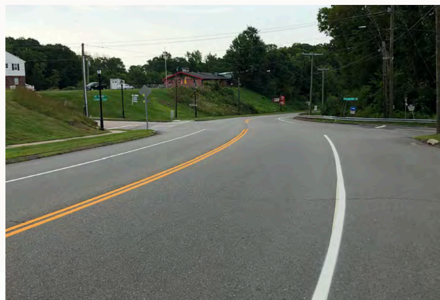
Horizontal and vertical curvature along CT-149 (Falls Road) looking west. Source: VN Engineers
