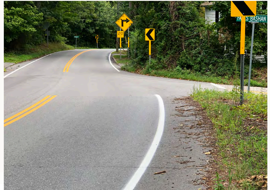
Horizontal and vertical curvature along CT-149 (Falls Road) looking north. Source: VN Engineers
