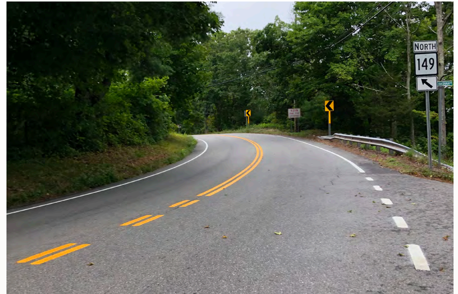
Horizontal and vertical curvature along CT-149 (Falls Road) looking east. Source: VN Engineers
