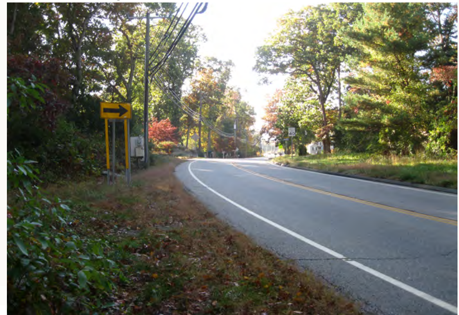
Reverse curve one-direction large arrow south of the intersection. Source: VN Engineers
