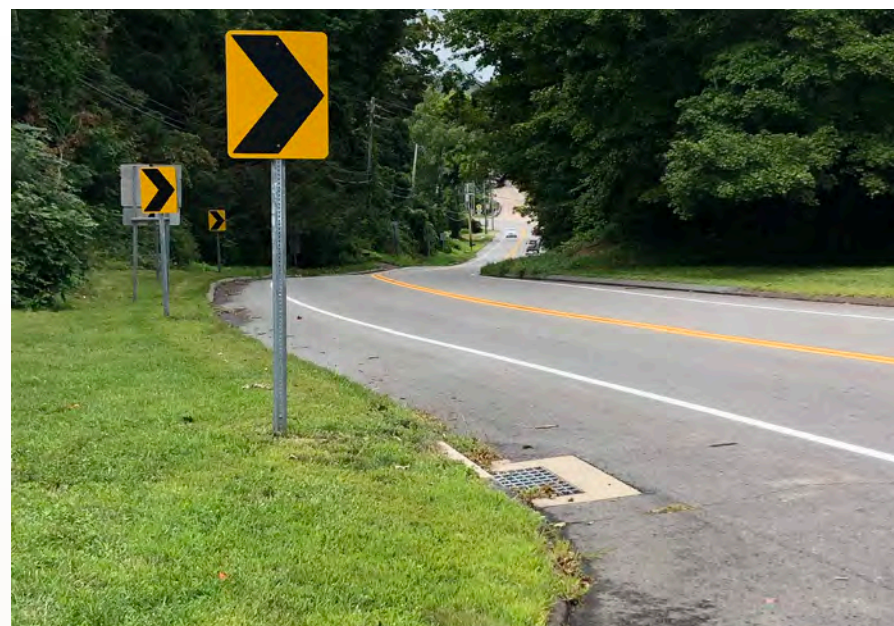
Horizontal and vertical curvature along CT-149 (East Haddam Moodus Road) looking west. Source: VN Engineers
