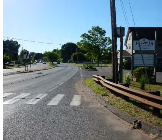
Non-ADA compliant pedestrian accommodations at the intersection of Route 66 and Airline Avenue
