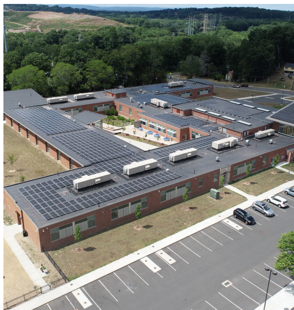
Figure 15: Roof-mounted solar panels at Verplanck Elementary School in Manchester.
